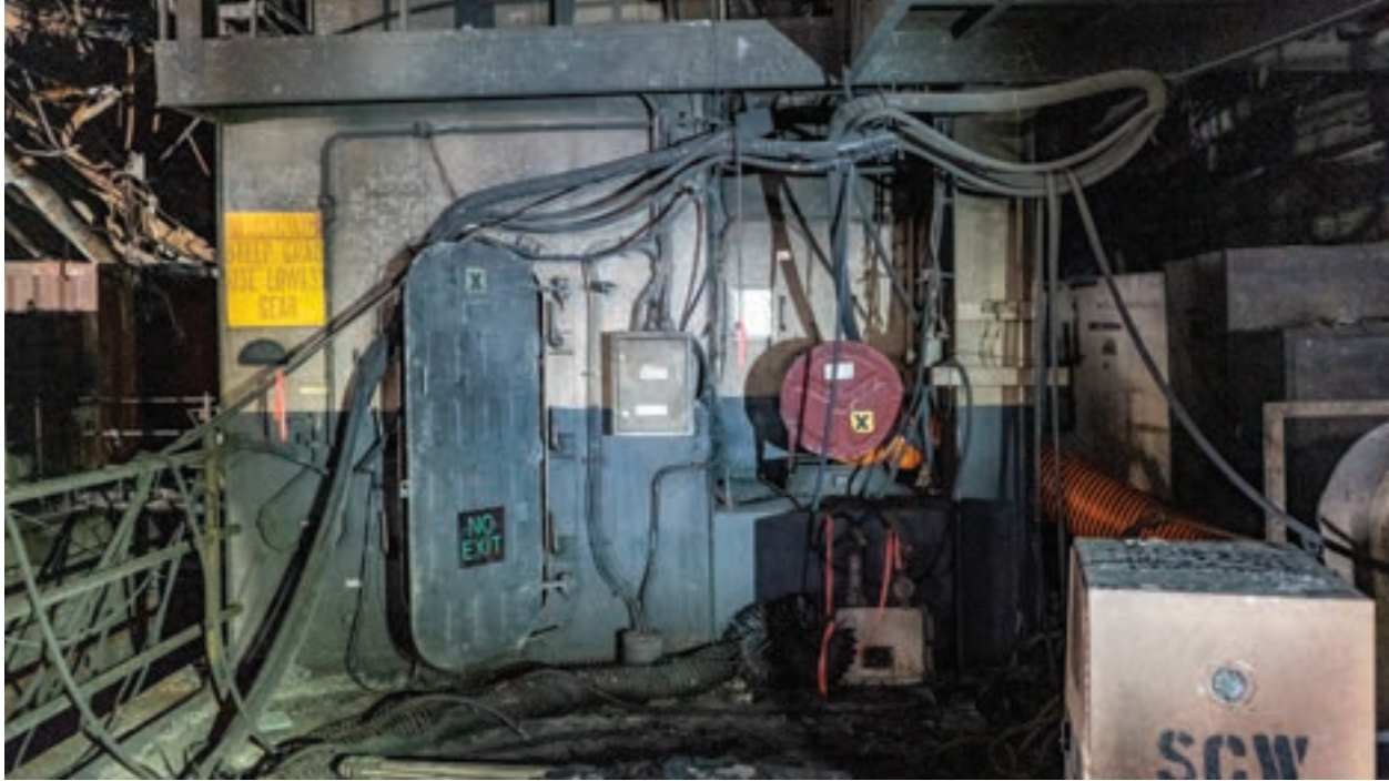
Figure 29, Still photo of AFFF push-buttons for sprinkler groups 15 and 16 serving Lower V (16 on left; 15 on right). These push-buttons are in Upper V amidships. An open hatch obstructs visibility of the push-buttons.
