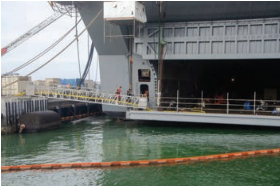
Figure 18 shows the stern gate brow, which was landed at approximately 0211 on 13 July 2020.
