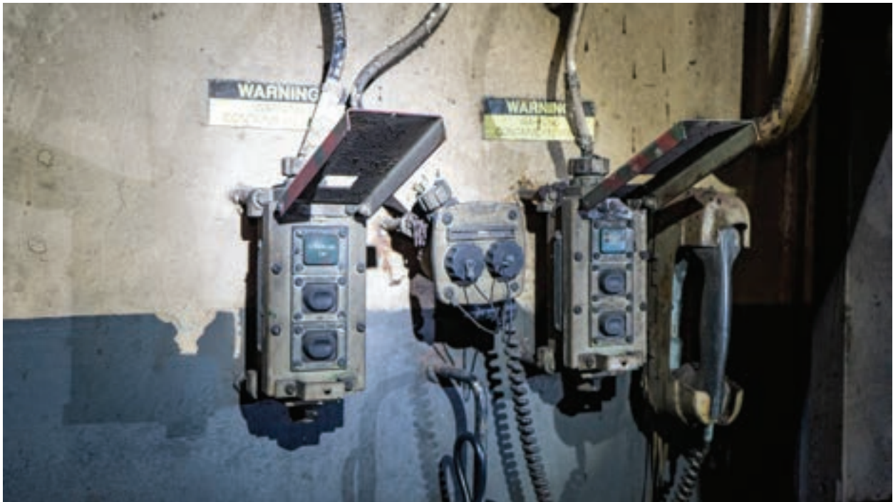
Figure 32, Still photo of AFFF push-buttons for sprinkler groups 15 and 16 serving Lower V with covers open (16 on left; 15 on right). These push-buttons are in Upper V amidships.
