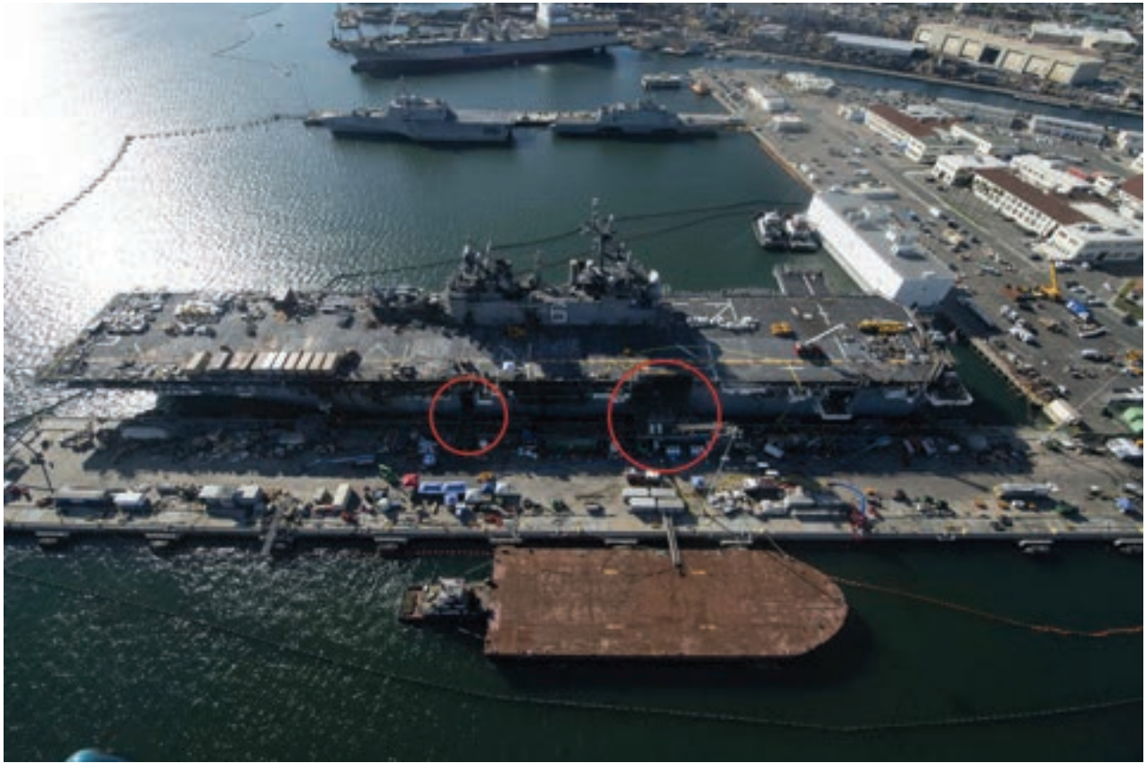
Figure 5 is a photograph of BONHOMME RICHARD with the sideport door/port ACE identified.
